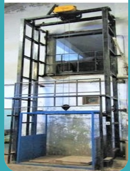
Wire Rope Goods Lift Capacity -200 To 2000 Kgs Lifting Height -50 Feet
